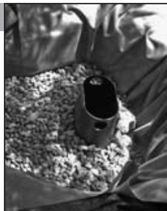
Fig. 25 Add gravel into the basin.
