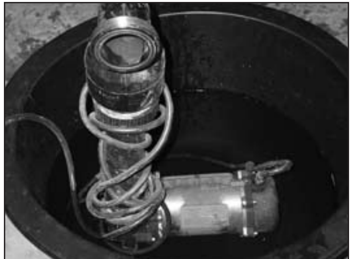
Fig. 51 The water in the bucket will prevent the pump seals from drying and cracking.
