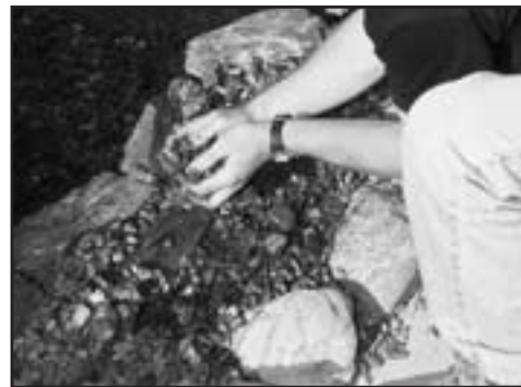
Fig. 47 Hide the exposed liner with gravel and mulch.
