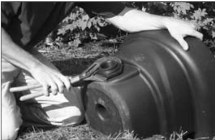
Fig. 4 Attach bulkhead fitting.
