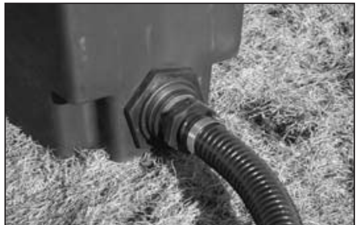
Fig. 7 Finished Bulkhead Assembly.
