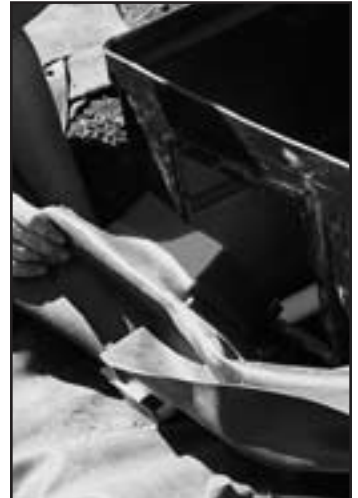
Fig. 24 Carefully replace the skimmer faceplate into the silicone lined opening.
