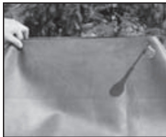
Fig. 33 Poke holes in the liner all the way through to the inside of the filter box.
