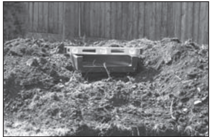
Fig. 10 Soil backfilled around the MicroFalls® helps hide the filter and creates a planting berm.
