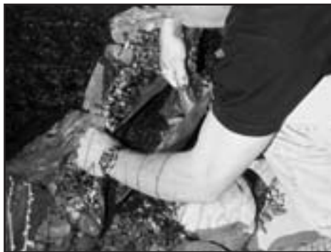
Fig. 46 If you find the leak, pack soil beneath the liner to raise the edge.
