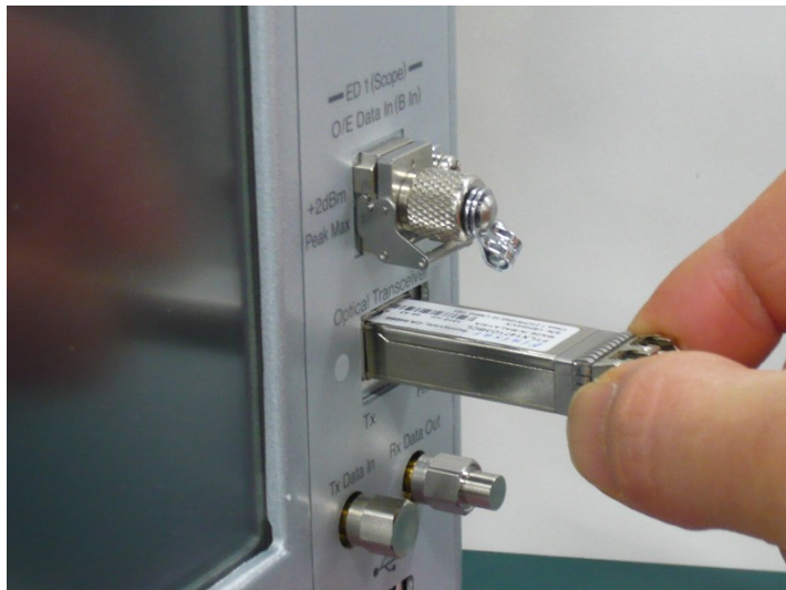
Figure 2.8.1-1 Installing Optical Transceiver
