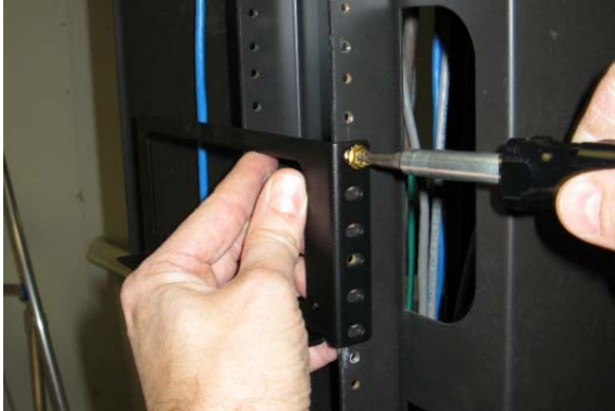
Figure 21: CX II/CXi II Controller Rack-Mount Installation - Attaching Brackets to Rack Frame
