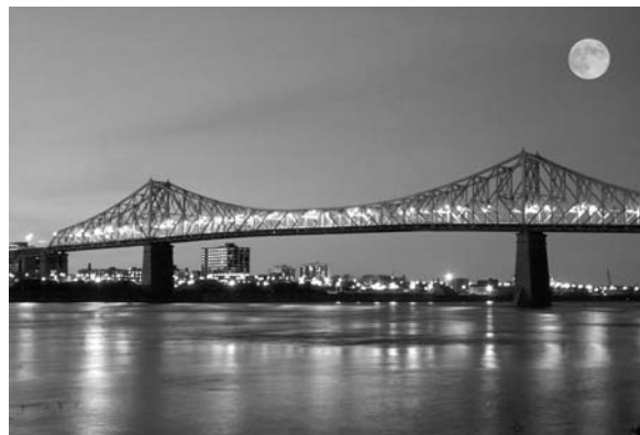
Jacques-Cartier Bridge, Montreal, Canada: a cantilever bridge that incorporates a supporting steel truss structure.
