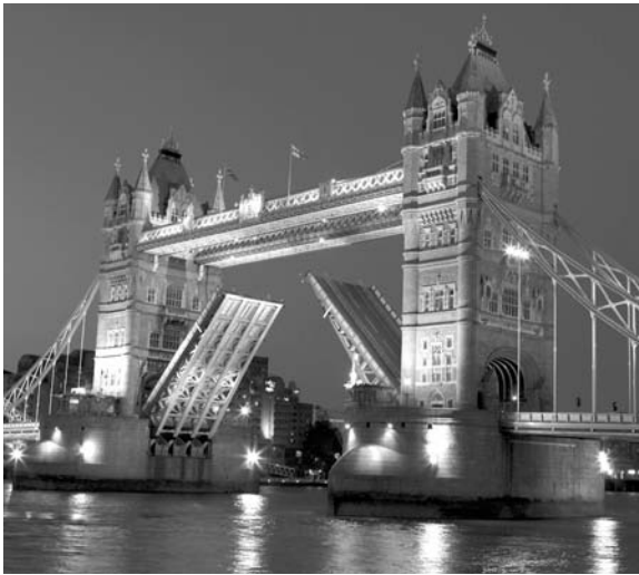
Tower Bridge, London, England.
