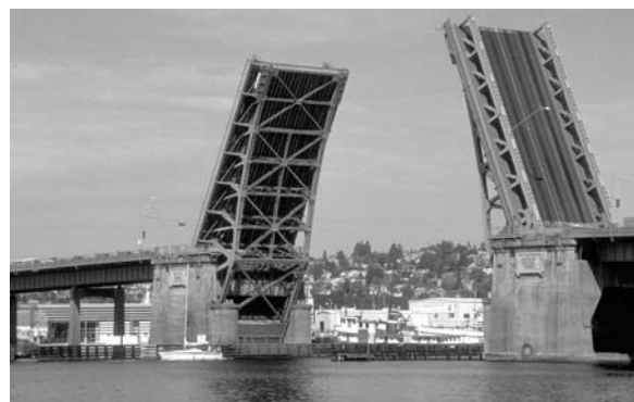
A bascule bridge opening for shipping
