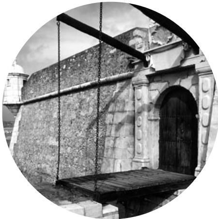
A castle drawbridge A drawbridge is a variation of a bascule bridge. Both types of bridges use the principle of the lever to operate.
