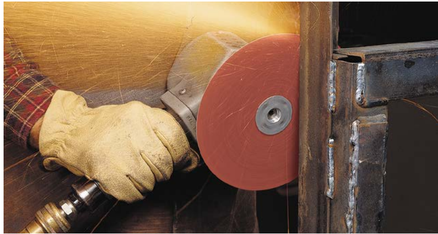
Weld spatter clean-up: 3M™ Fibre Disc 782C
