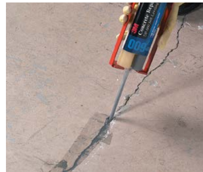
Fix cracks, spalls, and breaks in concrete:
