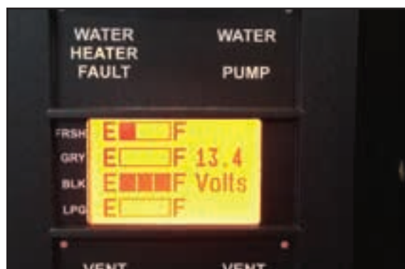
Figure 13-5: Water pump switch
