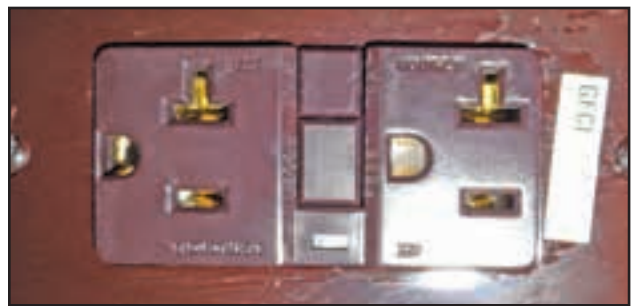
Figure 9-8: GFCI receptacle
