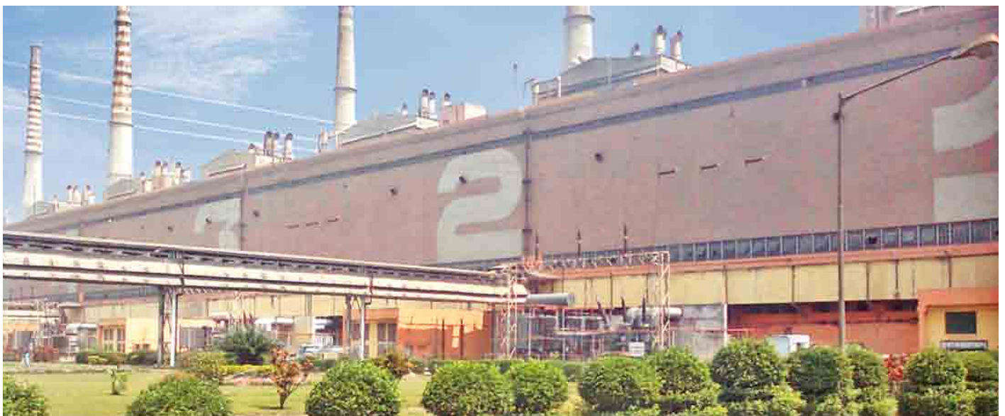
NALCO's Angul smelter produces up to 345,000 tons of aluminum a year, an increase of 50 percent on the previous capacity of 215,000 tons. The site's captive coal-fired power plant comprises ten 120 MW units, two of which are new.
