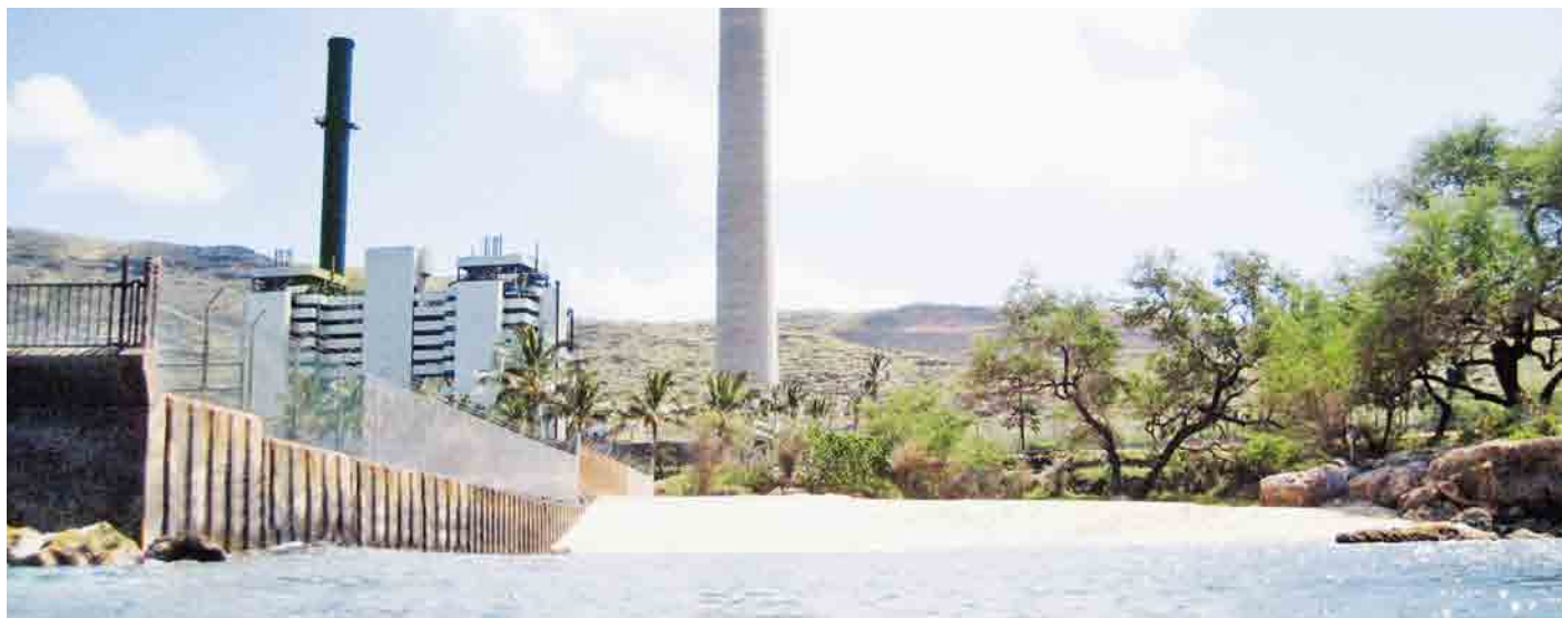
Kahe power plant, Hawaii
