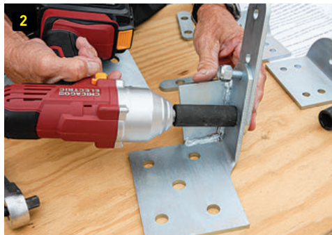
(1) Trailers often come from the factory with shock angles that are too severe to be effective. (2) Using ½-inch carriage bolts and Nylock nuts, install the shock mount extensions for the Joy Rider assemblies and tighten firmly.
