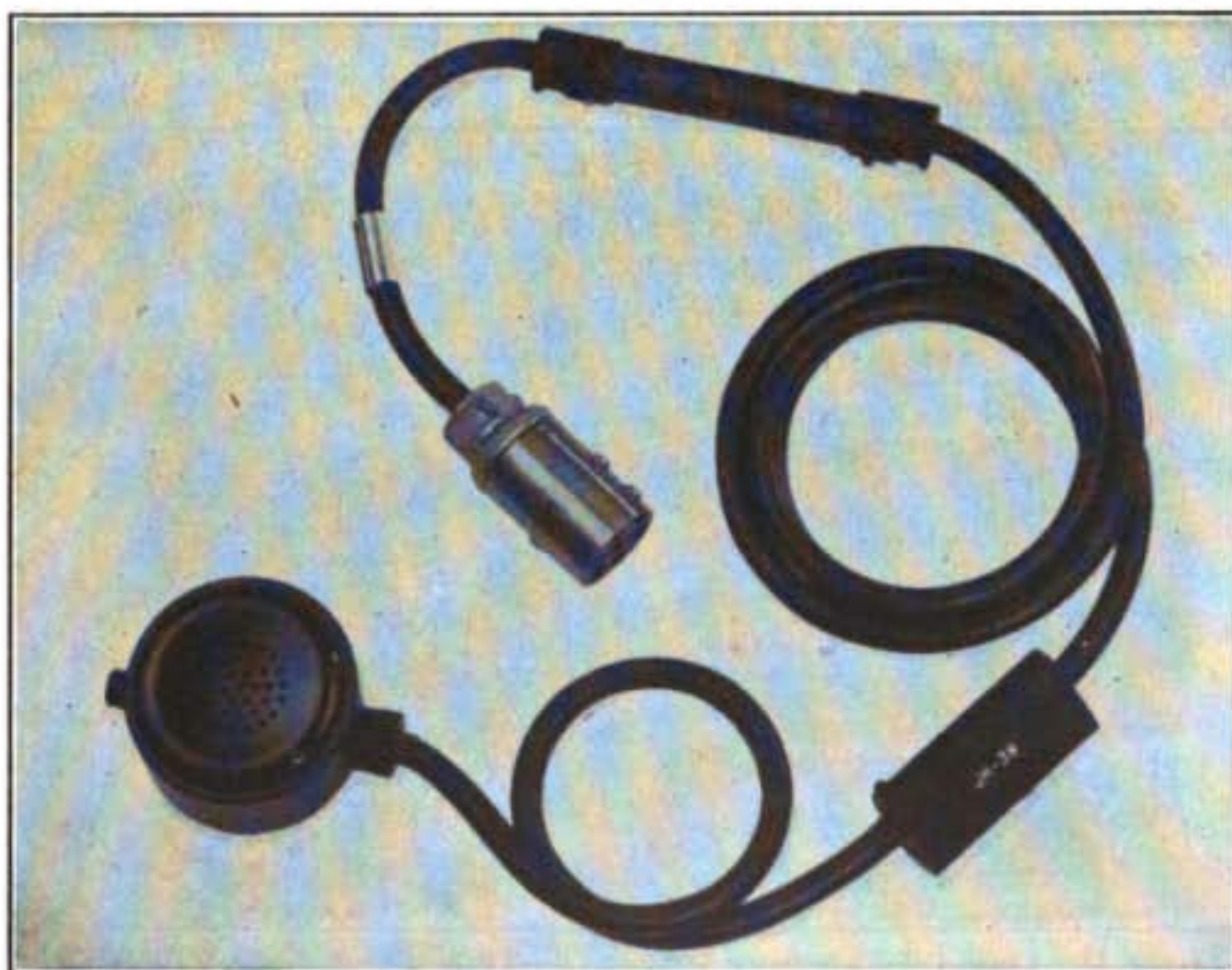
FIGURE 16.—Microphone T-24-E.
