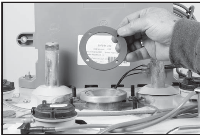
ORANGE SILICONE GASKET BETWEEN THE COMBUSTION BLOWER AND THE BLOWER FLANGE ON THE BURNER ADAPTER
