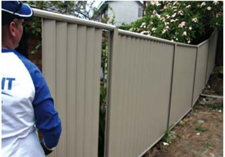
Lift top rail and place 1st sheet into bottom rail. Slide to end position.
