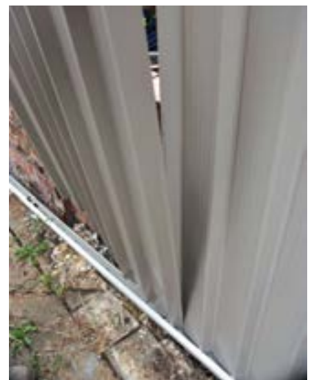
Place 2nd sheet into bottom rail, ensuring there is sufficient overlap.
