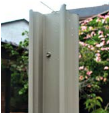
Use stringline to set post heights.
