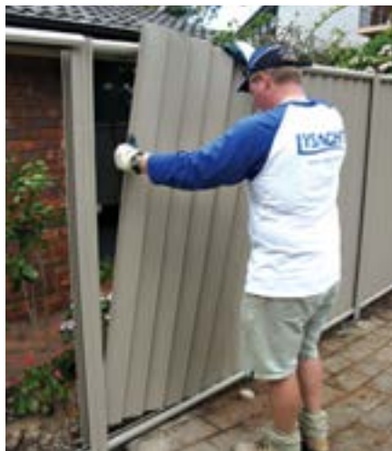
Position last sheet. Gentle force can be used.
