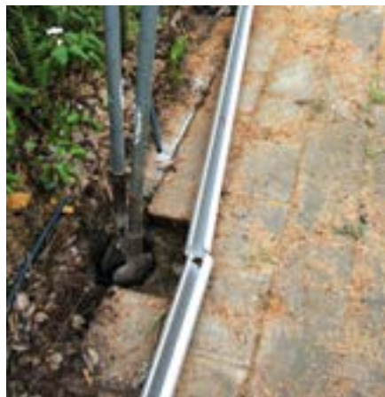
Lay the rails along the string line to determine positions of posts.
