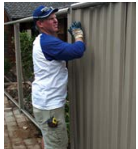
Lift top rail and rotate until infill sheet slides into rail. Tap top rail down into position.
