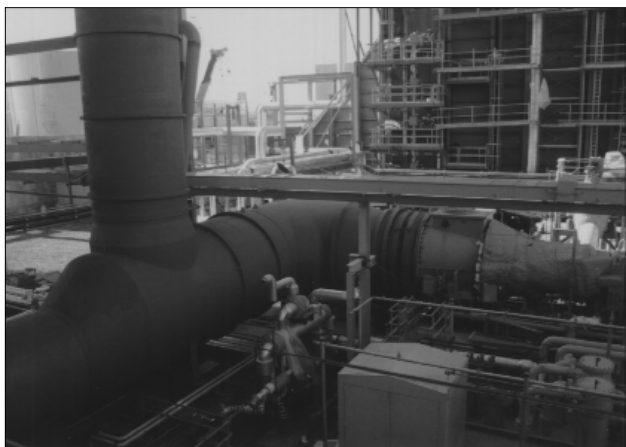
Figure 15. Axial exhaust steam turbine in air condenser application
