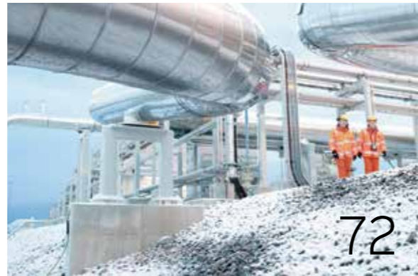
Process module engineering
