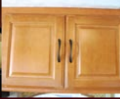
Raised Panel Cabinetry
