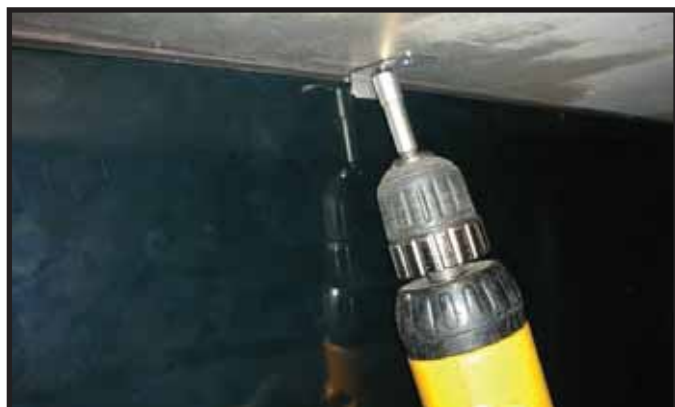
Figure 9. Fastening Angle Tab to Secure Inner Back Panel.
