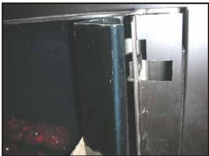
Figure 9. Installing Outside Corner Trim Piece onto Clip.
