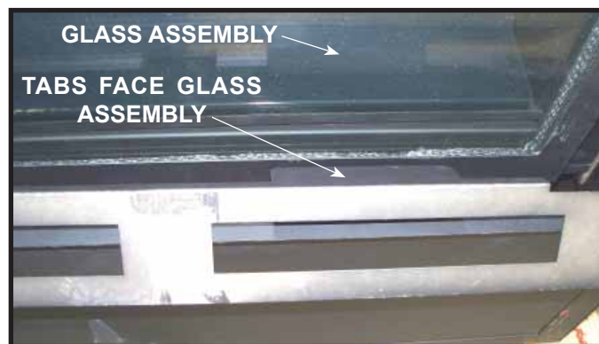
Figure 12. Positioning Porcelain Access Panel.
