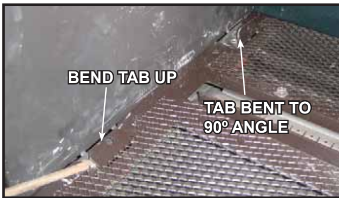
Figure 7. Bend Tabs Up to a 90 Degree Angle.
