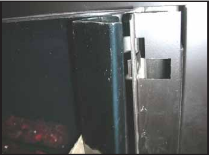
Figure 16. Installing Outside Corner Trim Piece onto Clip.
