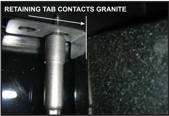
Figure 10. Placing Outer Corner Granite Trim Piece.
