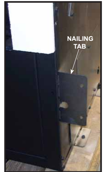
Figure 6.4 Nailing Tabs Installation Position
