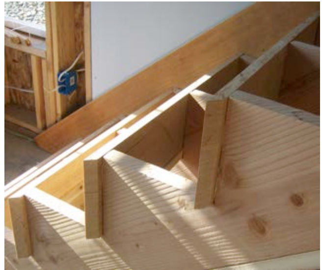
Mitred risers on open cut stringer. Used in conjunction with the bracketed strings.
