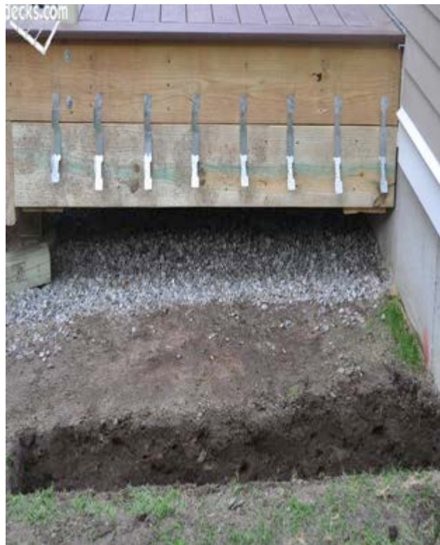
Brackets secured to deck side face and foundation prepared for concrete.
