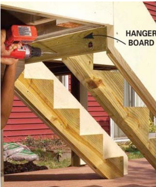
Stringers screwed to hanger board.
