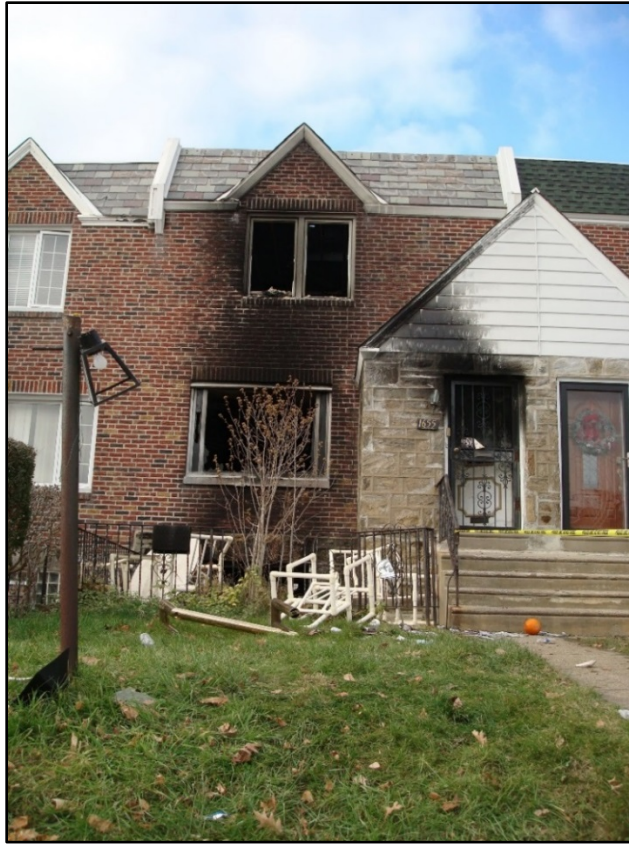
Photo 1. Front of row house. (NIOSH photo.)
