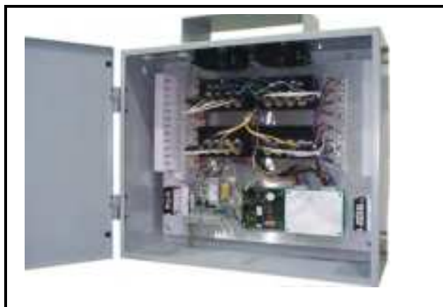
Figure 2-17 - PMAC II Anti-Sweat Control Panel
