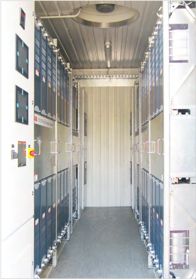
Two 1250 kVA PCS100 SFCs installed at Viktor Lenac shipyard
