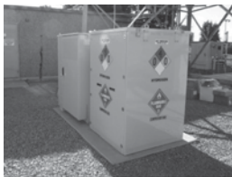
Figure 3: Actual Fuel Cell and Hydrogen Storage Cabinet Installation
