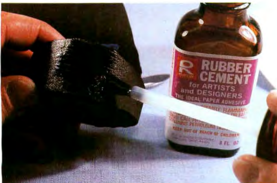
Photo 4: Apply rubber cement to the outside of the wedge-shaped piece of pipe insulation.
