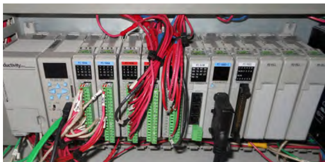
IMAGE 2: Productivity2000 PLC controls water treatment skid
