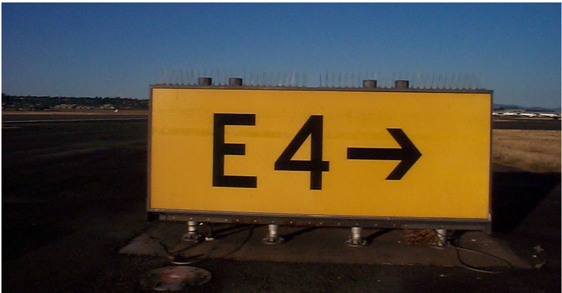
Runway Exit Sign on Runway 3/21
