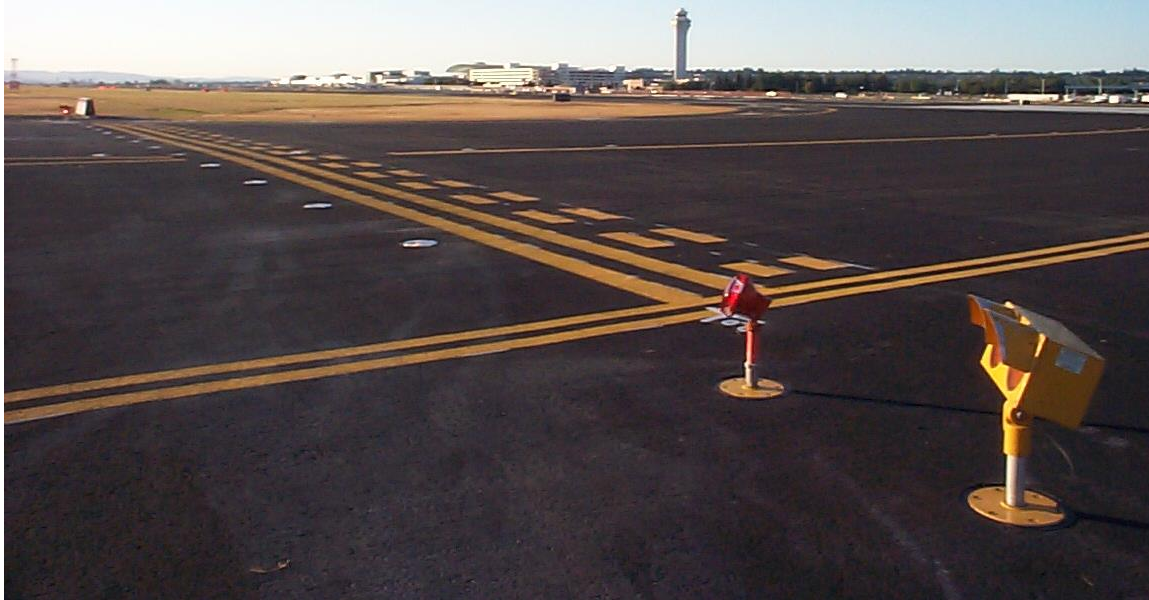
Runway Hold Bar Markings with Runway Guard Lights and Stop Bar Lights
