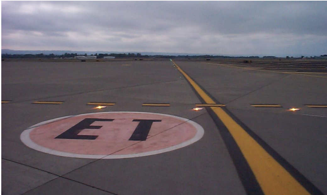
Geographic Position Marking with Clearance Bar Lights
