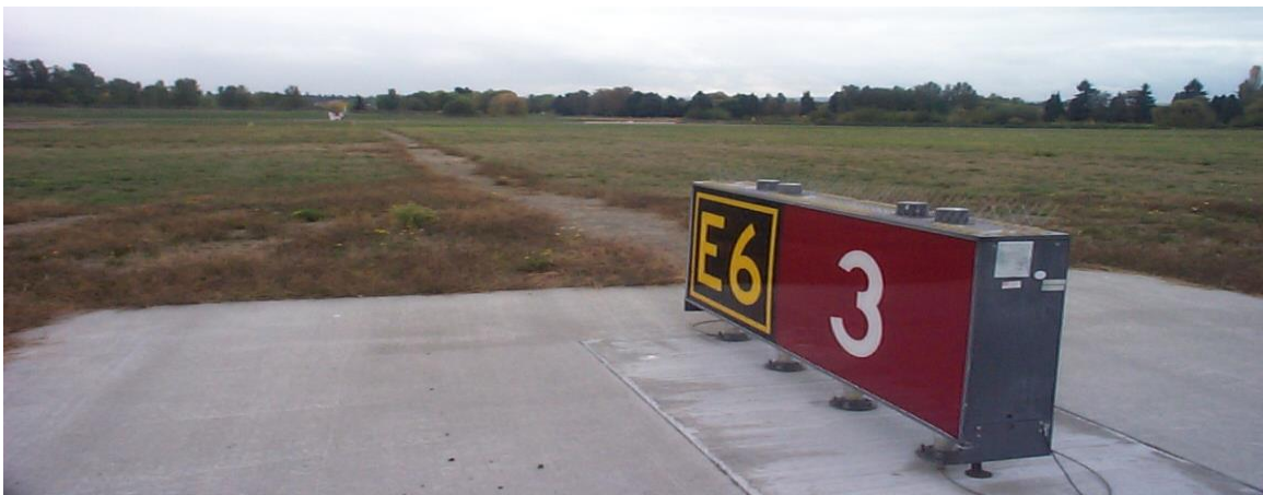
Line Denoting Runway Safety Area Boundary
