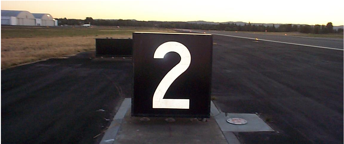
Distance Remaining Sign
