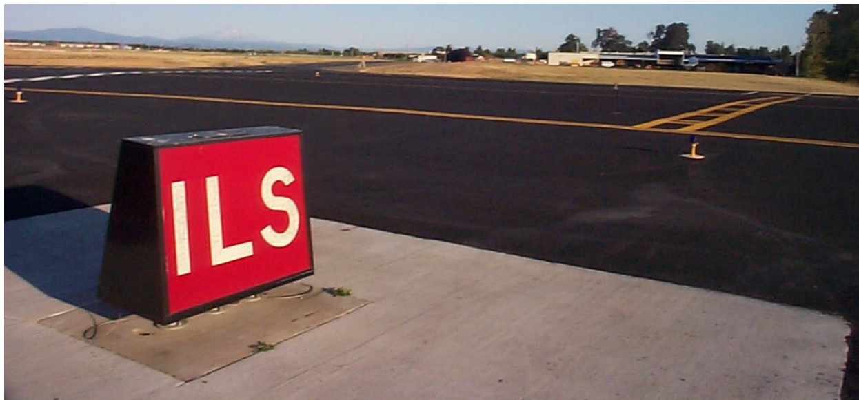
ILS Hold Position Sign and Hold Position Markings
