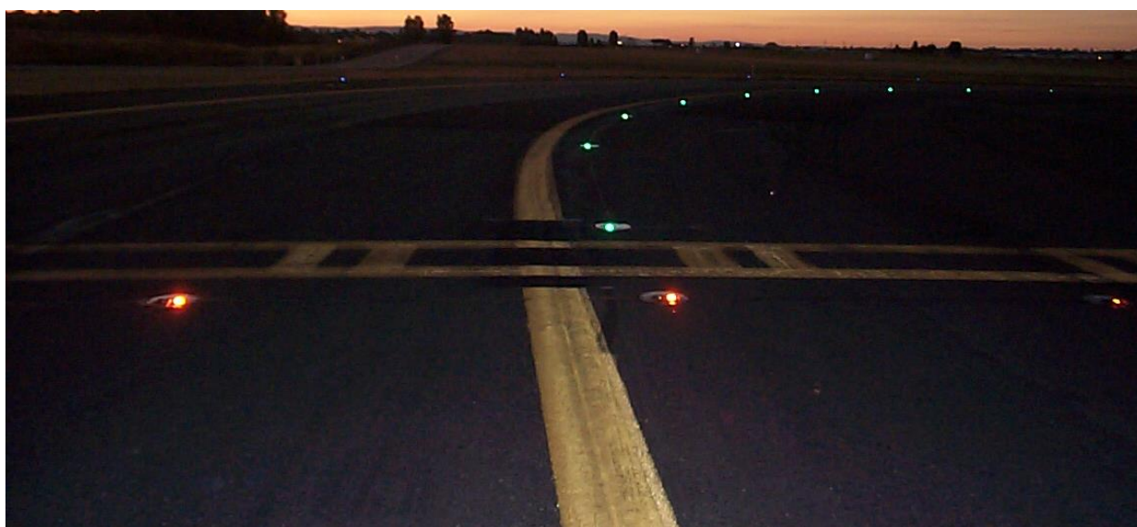
ILS Hold Position with in-pavement lights
