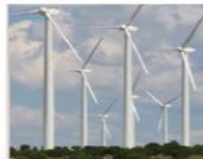
Aragonne Mesa Wind 90 MW
