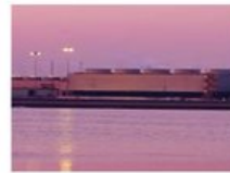
Salton Sea Geothermal 10 MW
