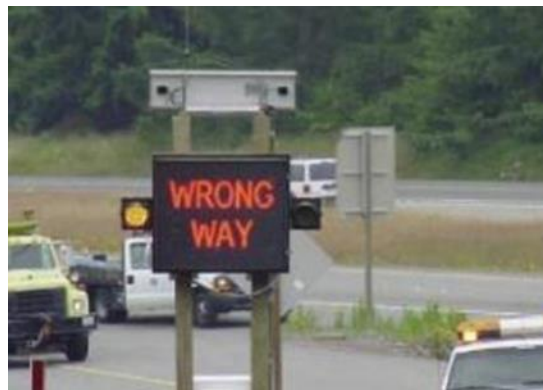
Figure 5.6.16–5: Example of LED-Enhanced Wrong-Way Signage
