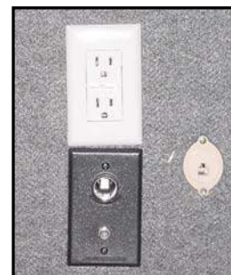
Figure 7-10. 12 VDC Receptacle (black)
