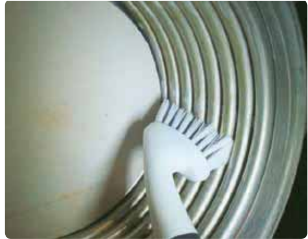
Figure 146 Cleaning the heat exchanger
