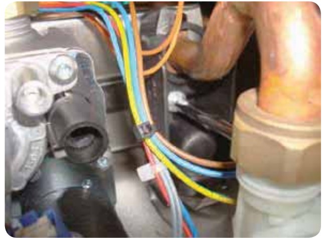
Figure 153 Removal of flat plate heat exchanger (screw on right side) (Combi Only 80/120 shown)
