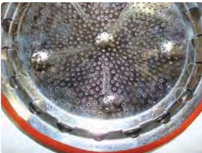
Figure 142 Inspecting interior and cleaning the burner
