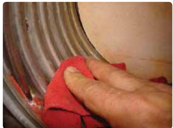
Figure 147 Cleaning the heat exchanger
