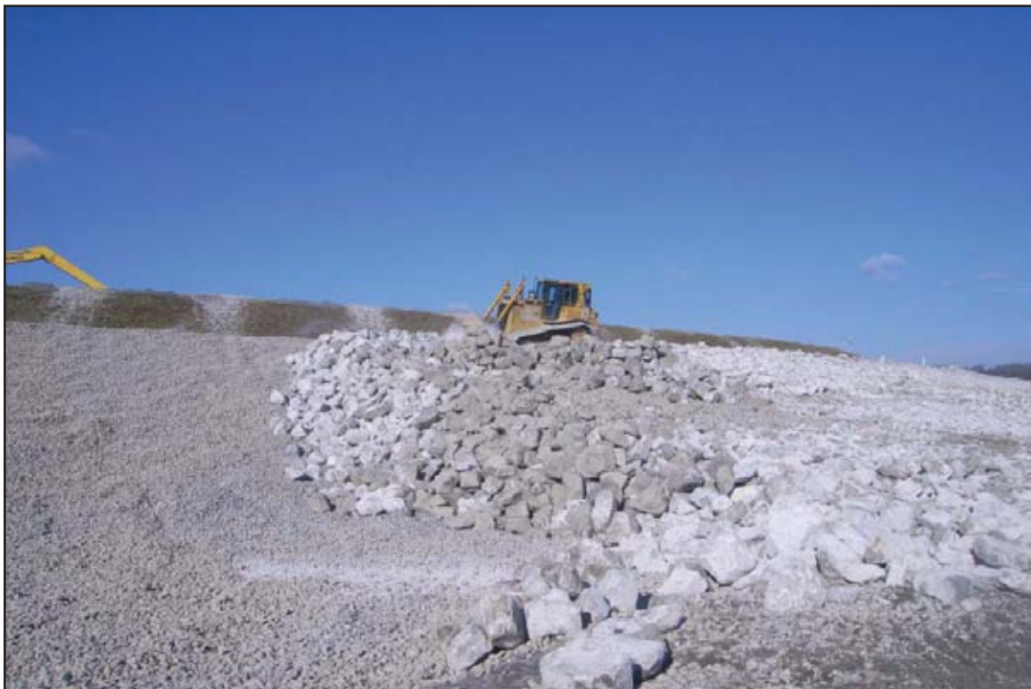
Placing riprap on top of gravel material. December 27, 2009.
