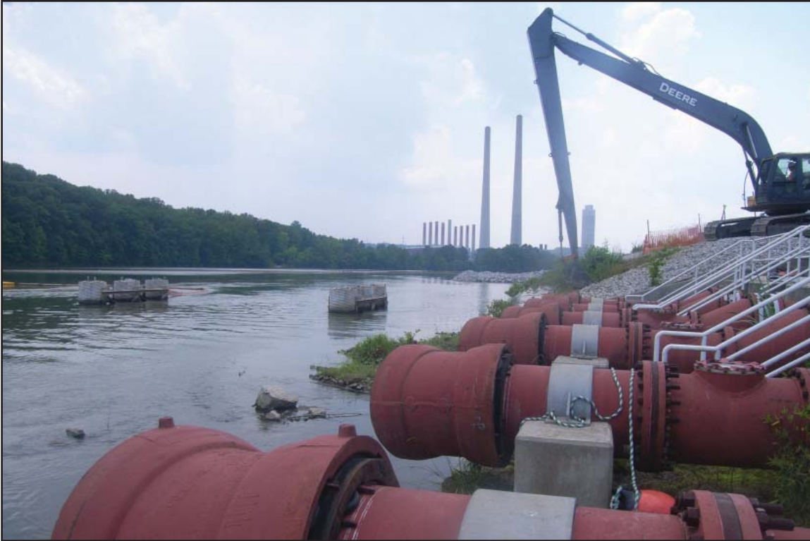
Old diffuser removal. June 11, 2011.
