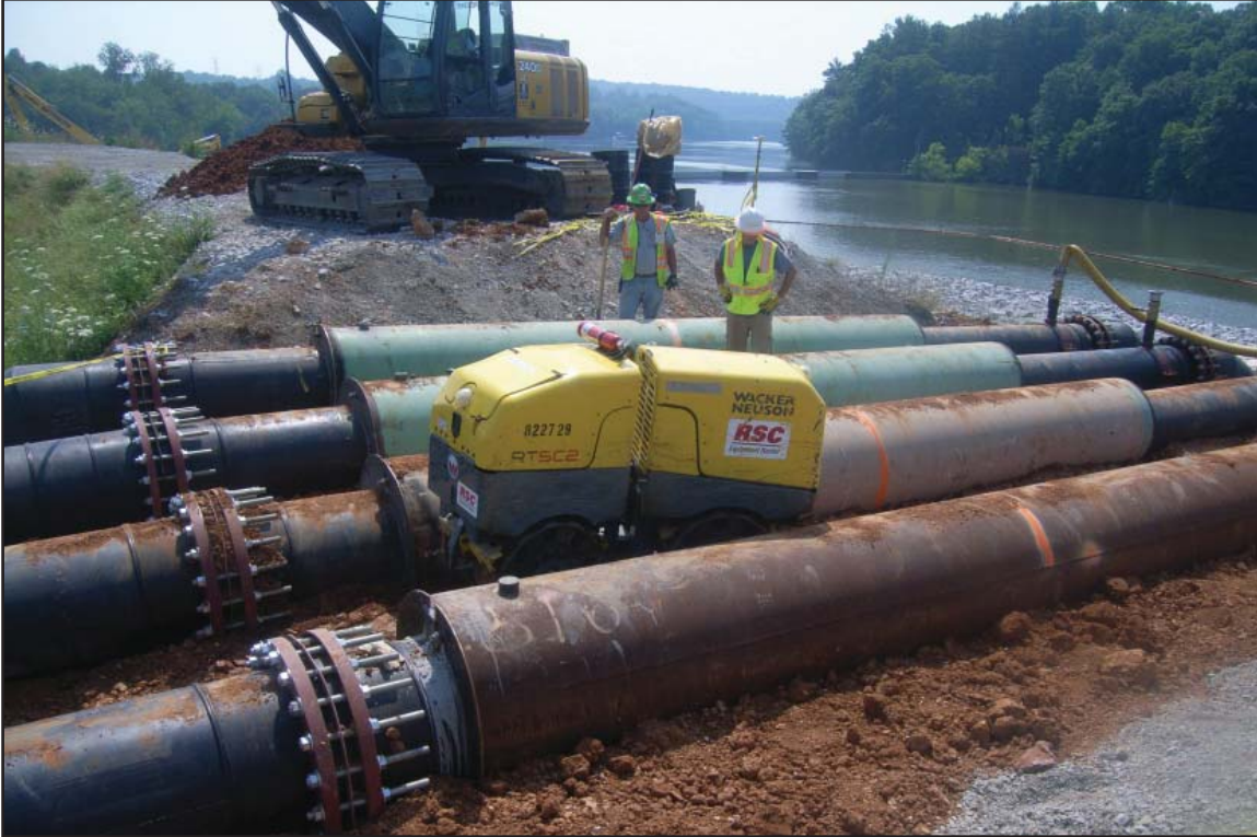
New siphon installation. June 7, 2011.
