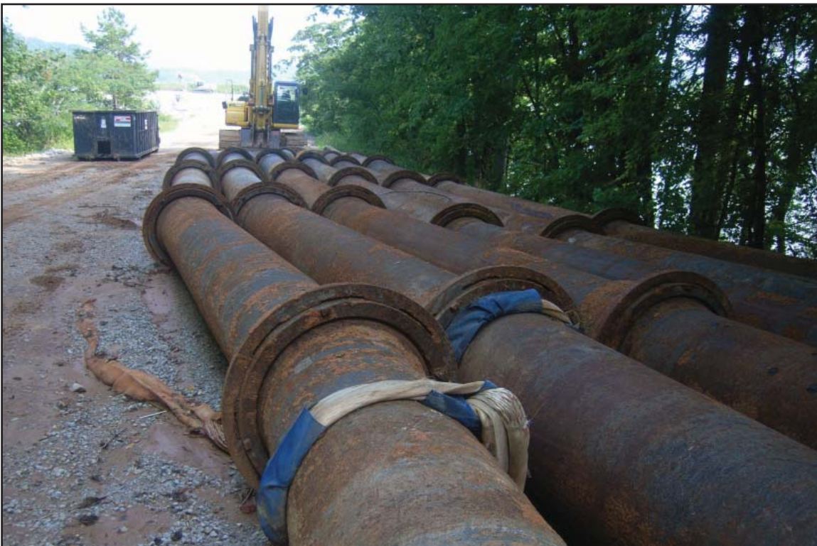
Old diffuser removal. July 19, 2011.
