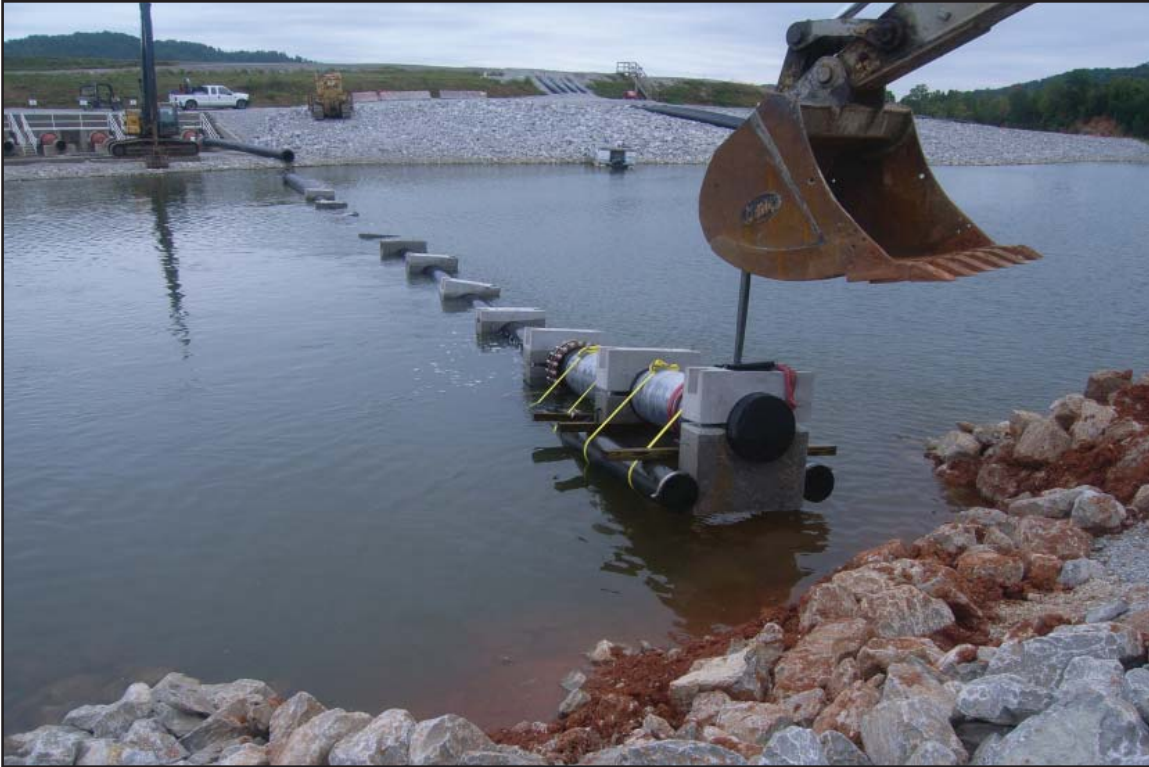
New diffuser installation. September 16, 2011.
