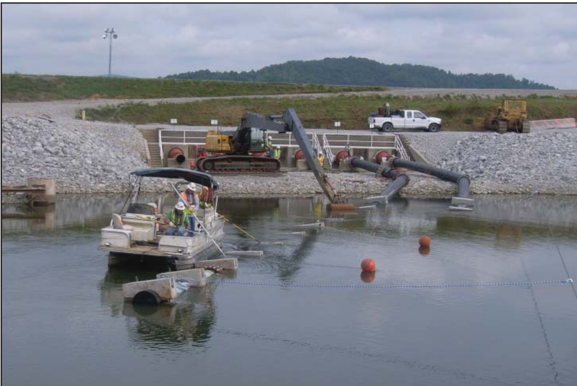
New diffuser installation. September 18, 2011.
