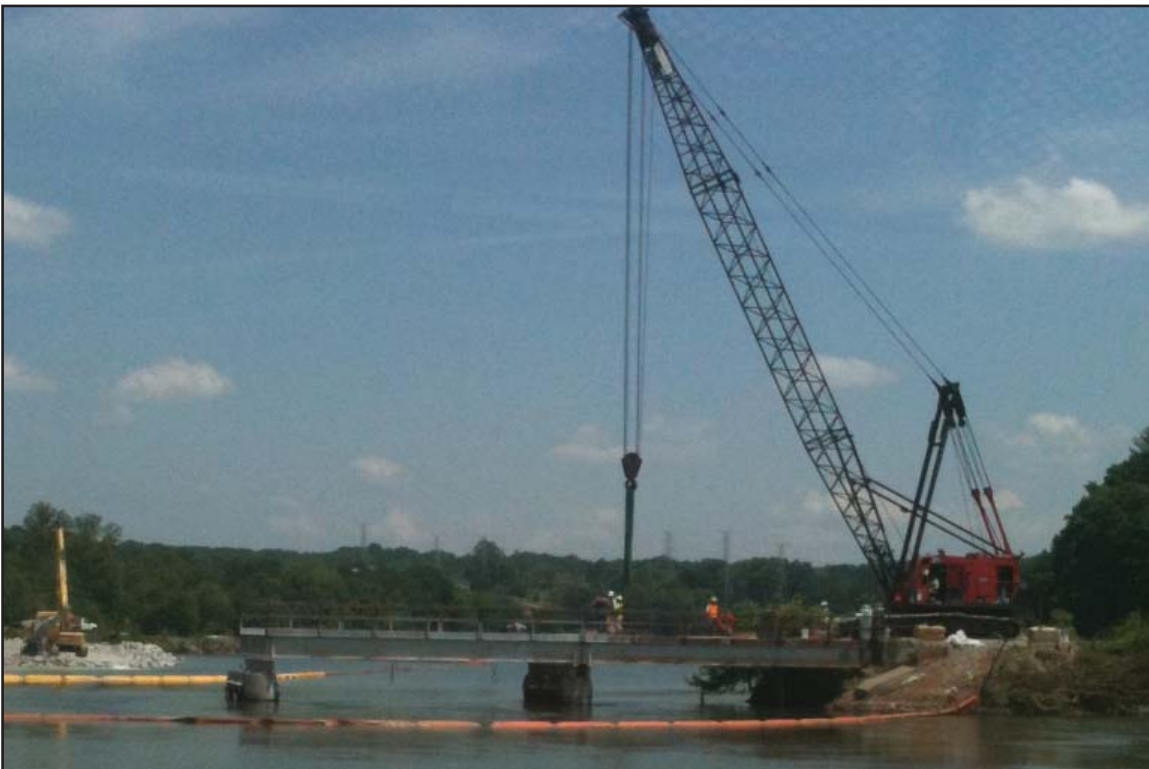
Bridge removal. May 2011.
