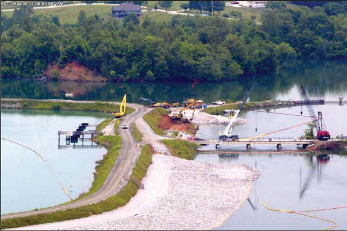
Bridge removal. May 6, 2011.
