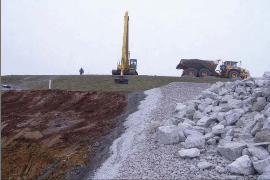
Excavation of subsequent panel next to a completed panel. February 12, 2010.
