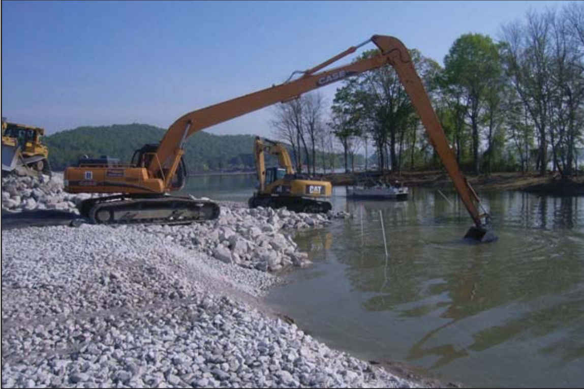
Below water excavation and sand, gravel, and riprap placement. April 23, 2010.
