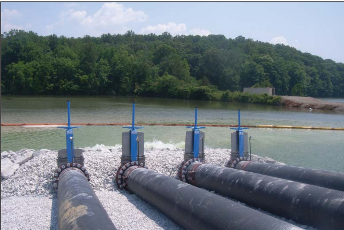
New siphon installation. June 7, 2011.
