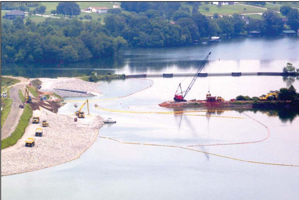
Causeway removal. July 5, 2011.
