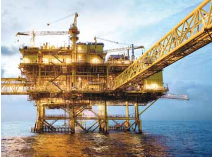
PB-KU-H Production Platform, Mexico for Pemex
