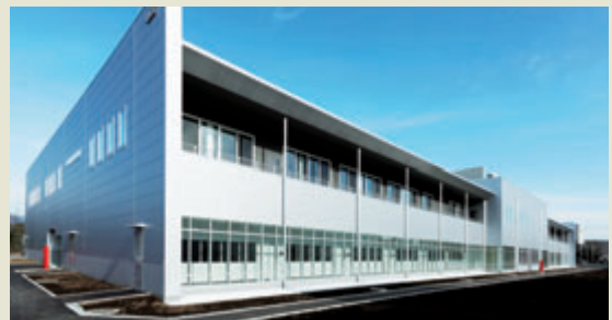
Customer Support and Training Center (Japan)
