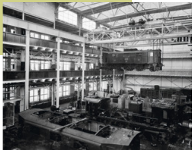
Expansion of the Dynamowerk – the locomotive assembly hall on the east side, 1913
