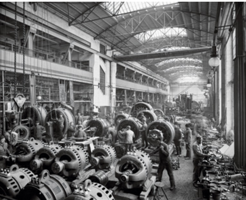
Products for Germany and the world – the motor department at the Charlottenburg plant of Siemens & Halske, 1899 (left), and the loading of oil-filled cables for Argentina at Gartenfeld cable plant, 1931 (right)
