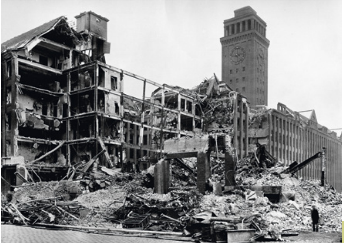
Signs of the war – Wernerwerk II partially damaged by bombings, 1944 (left) and damaged Dynamowerk, 1944 (right)
