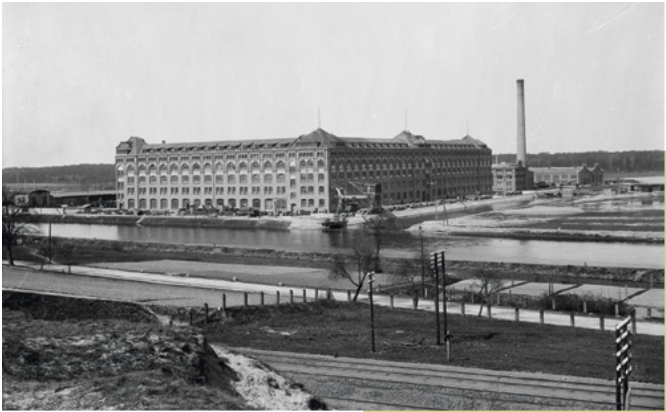
The nucleus of Siemensstadt – Siemens & Halske's new Kabelwerk on a canal branch of the Spree River, 1899
