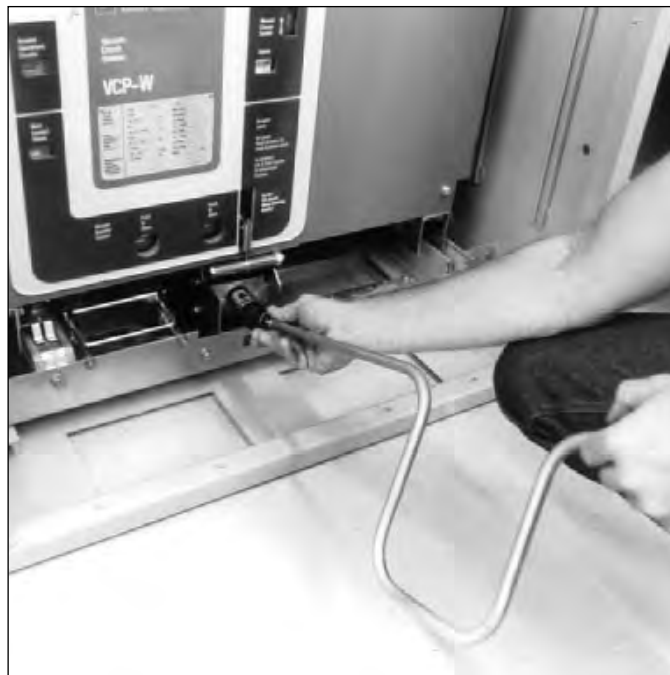
Figure 4-6 Engaging Levering-In Crank
