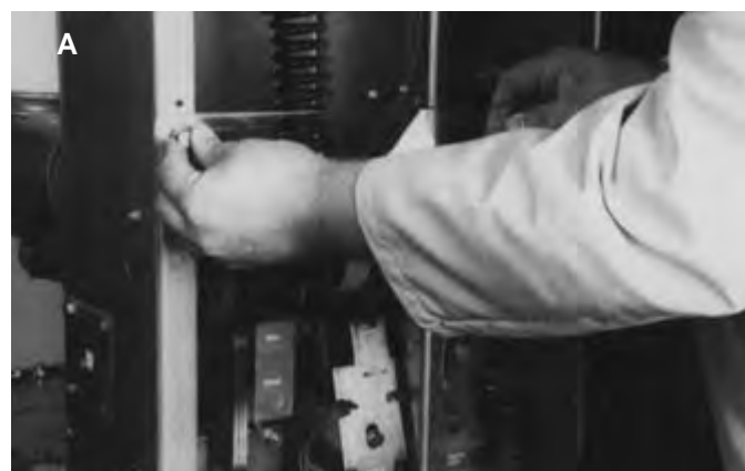
Figure 6-9 Attaching CloSure™ Test Tool at Hole “A”
