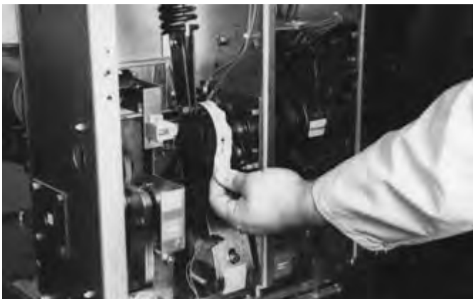
Figure 6-16 Remove Marked Masking Tape from Cam
