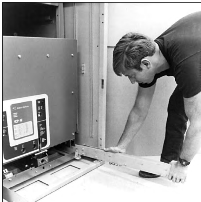
Figure 4-3 Engaging Extension Rails in a Lower Circuit Breaker Compartment
