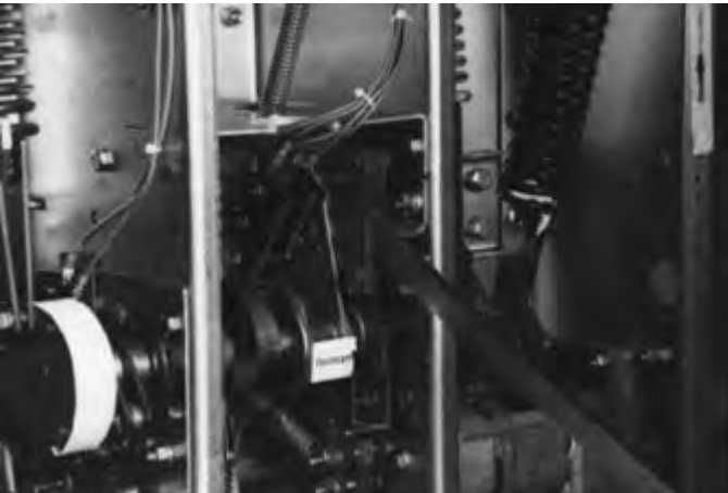
Figure 6-11 Manually Charging Closing Springs
