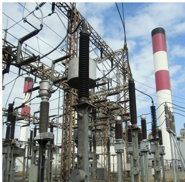
Is it safe to keep these 30 years old surge arresters for another 5 years?
