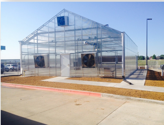
Birdville Center of Technology and Advanced Learning Green House Before
