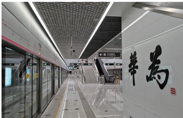
Huawei Station, Shenzhen Metro Line 10. Line 10 was one of the first metro lines in China with full 5G coverage and adopted Huawei's Urban Rail Cloud Solution.
