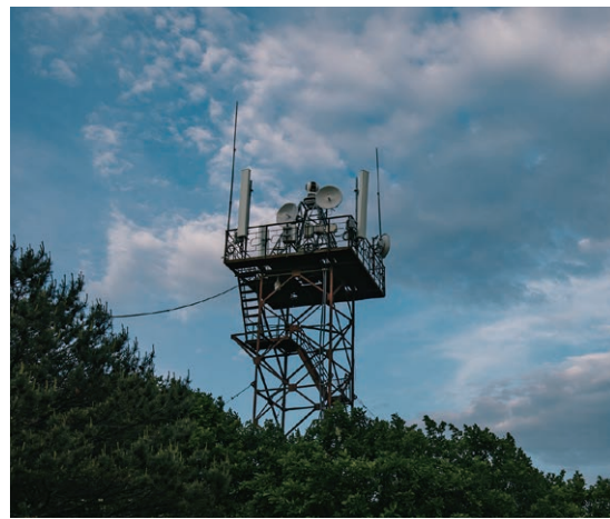
An LTE base station in the Northeastern China Tiger and Leopard National Park that reuses existing fire towers
