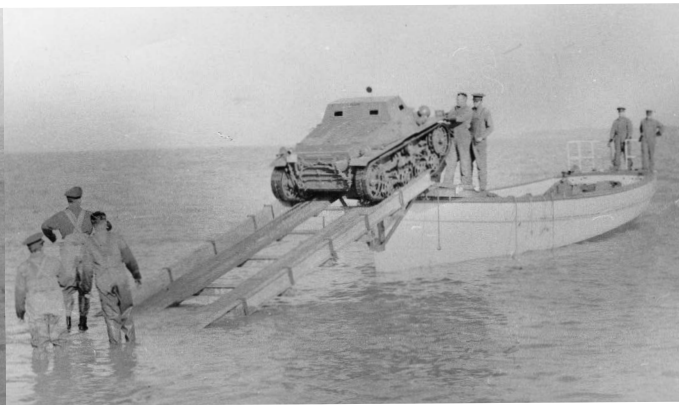
Below: A series of three shots showing the US Marine Corps practising amphibious landings using a Marmon-Herrington CTL-3 tank and a 50ft launch. For safety reasons the tank had to be reversed ashore.
