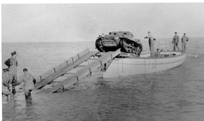
Below: A series of three shots showing the US Marine Corps practising amphibious landings using a Marmon-Herrington CTL-3 tank and a 50ft launch. For safety reasons the tank had to be reversed ashore.
