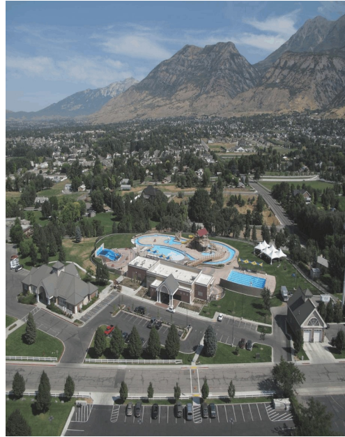
Aerial photo of Lindon City Aquatics Center
