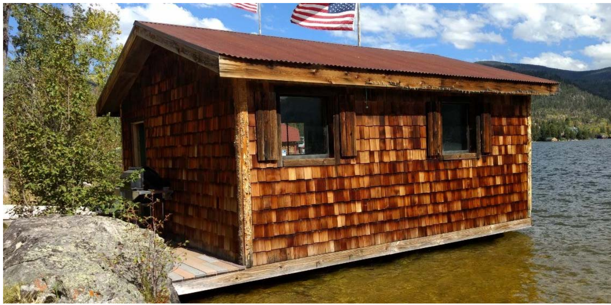
EXISTING BOATHOUSE - PROPOSED EXTERIOR MATERIALS TO MATCH EXISTING
