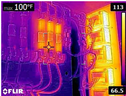
Check newly-installed electrical wiring
