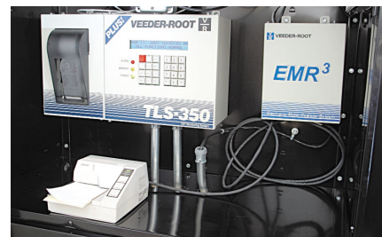
The EMR 3 can be connected to any Veeder-Root TLS series automatic tank gauge for enhanced fuel monitoring capabilities
