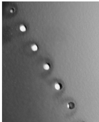
BLOCKED CARRYOVER PORTS
