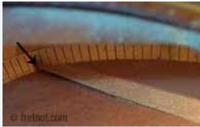
Loose Back Brace
