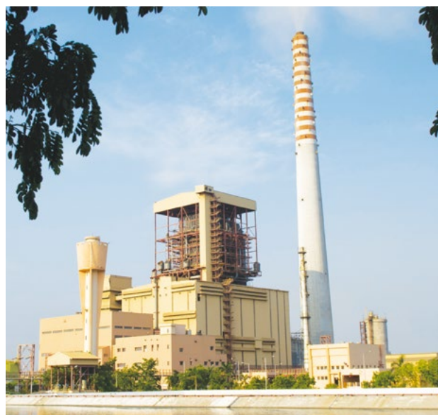
250MW TAQA Neyveli lignite-fired plant
