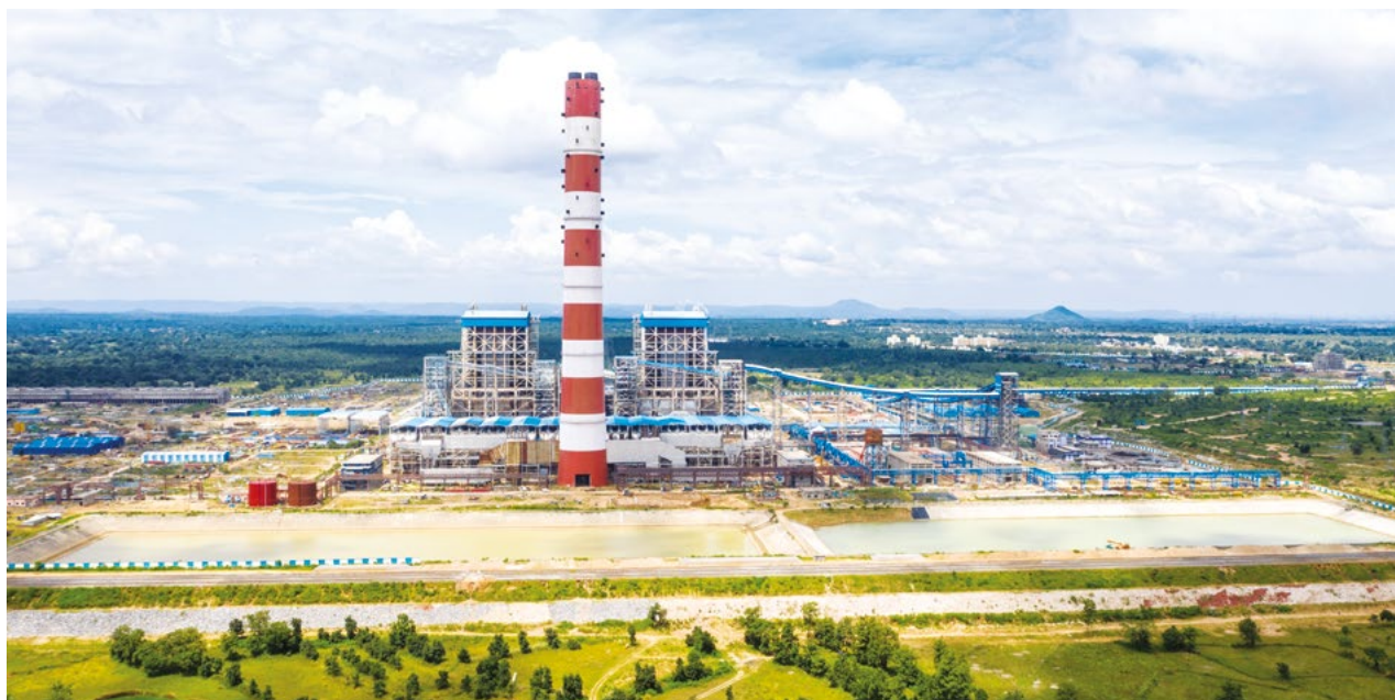
2X800MW NTPC Super Thermal Power Project, Daripalli, Odisha
