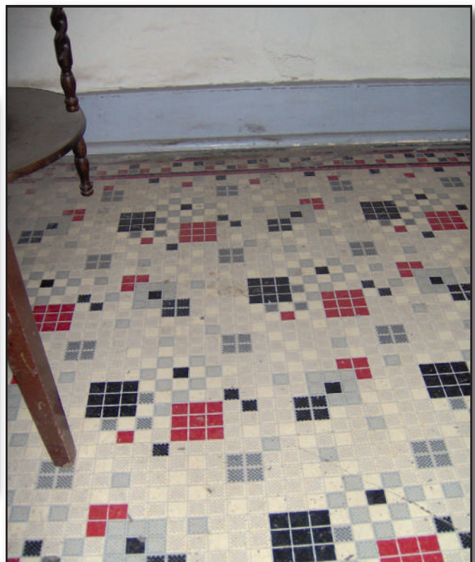
Figure 3—This linoleum flooring is holding up fairly well, but the printed pattern is scratched and worn.
