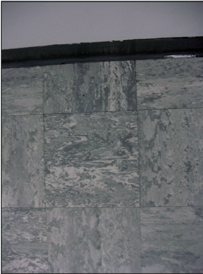
Figure 6—Although vinyl flooring can be manufactured in almost any pattern and color, this vinyl tile in the Intermountain Regional Office (Ogden, UT) is patterned to resemble gray-and-white marble.
