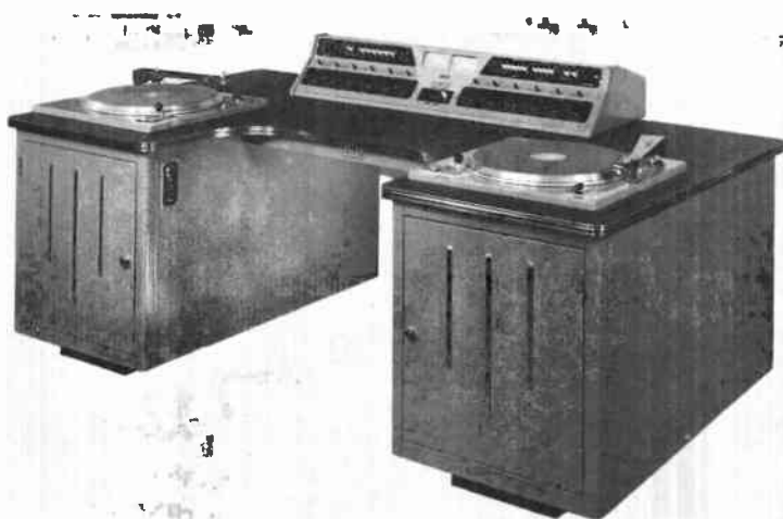
Fig. 5-1. Gates turntables and control room console.
