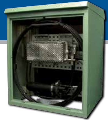
Fibernode Power Enclosure (Rear)
