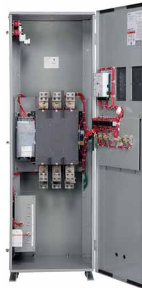
1200 A ATS with ATC-300+ Controller
