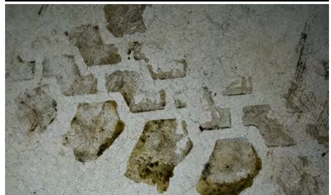
Vehicle treads mark the floor inside the Defender Dome at Minot Air Force Base, N.D., July 28, 2016. The 91st Security Support Squadron is specifically responsible for preventative maintenance inspections and troubleshooting, and everything from electrical repair to transmission replacement, on armored Humvees and Bearcats. (U.S. Air Force photos/Airman 1st Class J.T. Armstrong)
