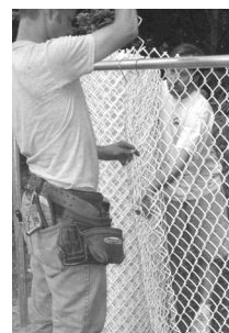
Weave additional rolls together to get the desired length. This is easier done laying horizontally, however it may also be done vertically.
