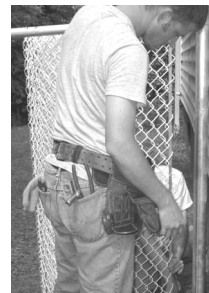
Stand up rolls on shorter stretches; use a pul-jak to stretch.
