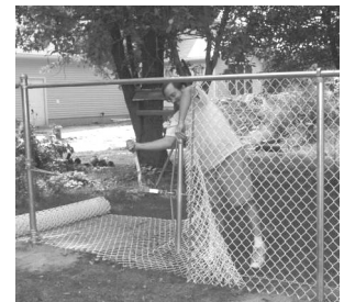
A come-a-long is required for longer stretches of chain link fence.
