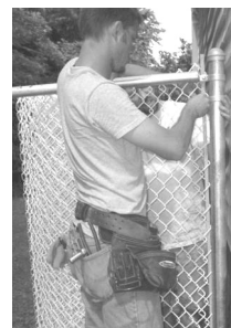
Hook up tension bands using 5/16" x 1-1/4" nuts and bolts. Adjust height before tightening.
