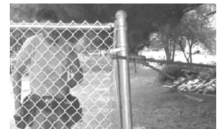
A pul-jak is the ideal tool for short stretches of chain link fence.
