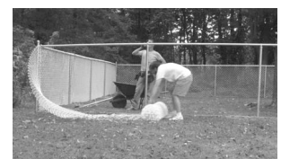
It is best to lay chain link rolls down flat for longer stretches.
