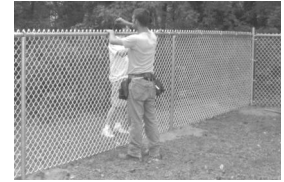
Be sure to center top chain link diamond on rail prior to tying.
