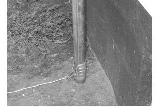
View of bottom brace band for bottom wire, and four tension bands for a 5' high chain link fence. View is from the inside of fence. Notice tension bands are offset so that the flat side is facing out.
