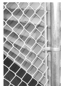
View of fence from inside: Notice flat side of tension band faces out, nut is on inside.
