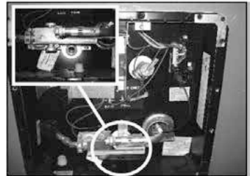
Fig 1: Water heater drain plug
